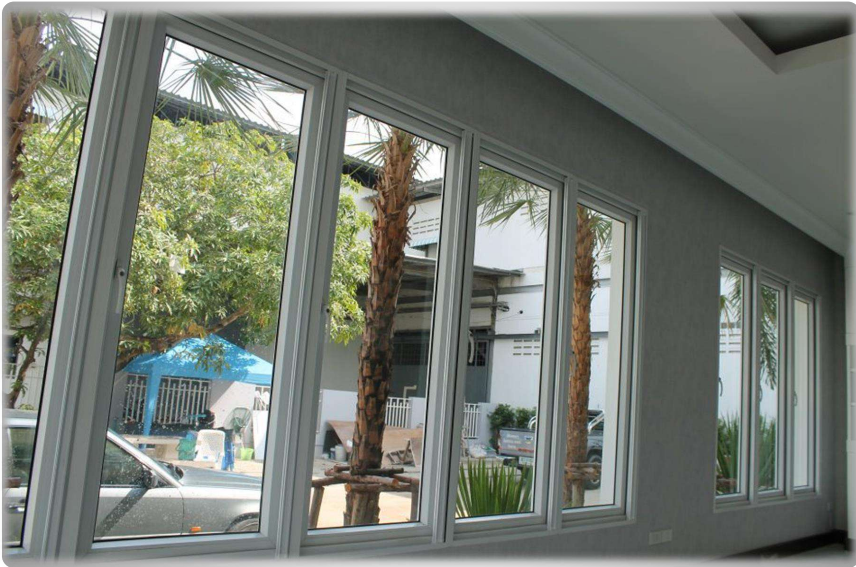
CASEMENT DOOR OUTSIDE OPENABLE
